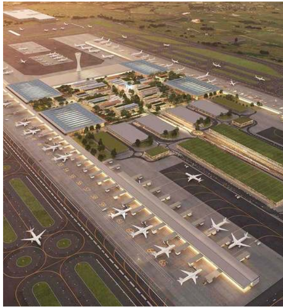
WESTERN SYDNEY AIRPORT COMPLETED
