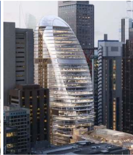
MARTIN PLACE NORTH COMPLETED
