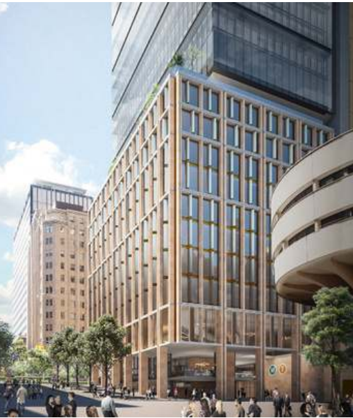
MARTIN PLACE SOUTH COMPLETED
