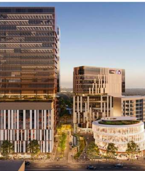
CIVIC PLACE LIVERPOOL COMPLETED
