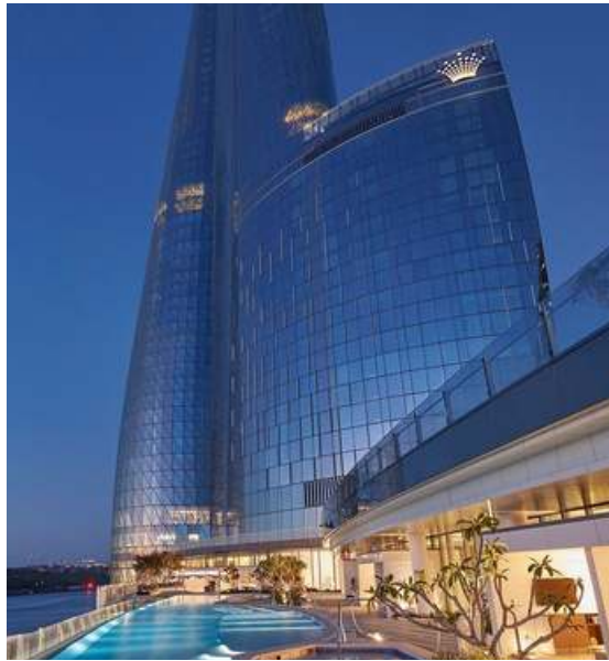
CROWN TOWERS SYDNEY COMPLETED
