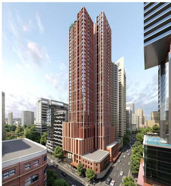
PITT ST SOUTH METRO COMPLETED
