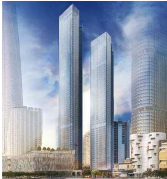
ONE SYDNEY HARBOUR COMPLETED
